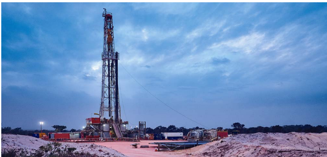
Above: Waitsia-3 appraisal well being drilled by Enerdrill Rig 3
