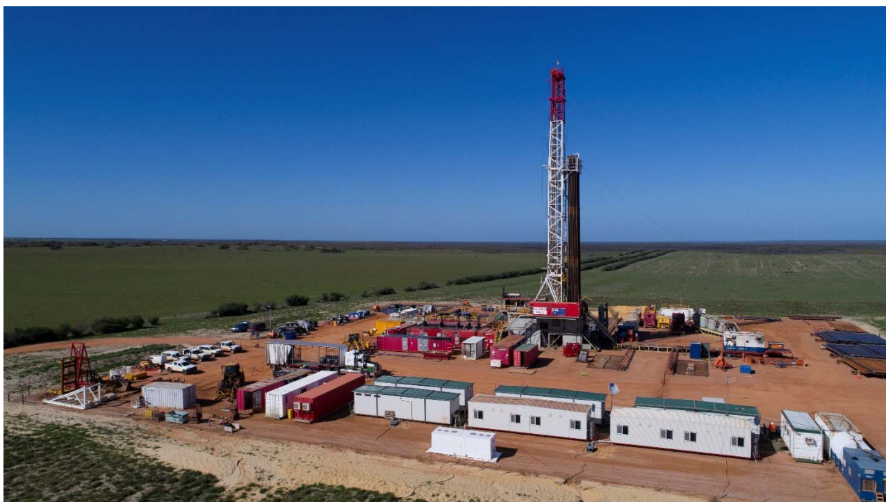
Above: Waitsia-4 appraisal well drilling, August 2017.
